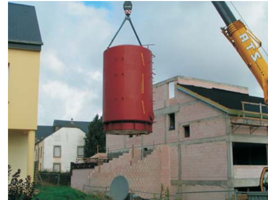
Fig 11: Installation of storage tank
