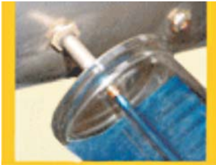
Fig 21: Heat pipe type collector
